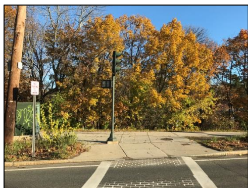
The “Don’t Walk” indication at the pedestrian signal across California Street does not work.
