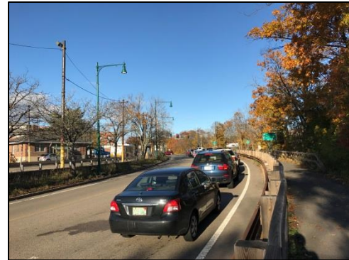
A horizontal curve on Nonantum Road may make it difficult for motorists to see the signal indications at the intersection.
