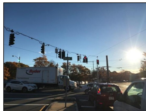
Crosswalk markings are not easily distinguishable from “Do Not Block Intersection” markings. Vehicles often stop in the crosswalks, forcing pedestrians to walk between queued vehicles.
